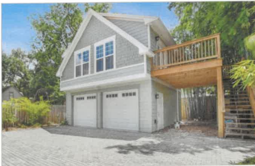
Figure 16: Elevated Accessory Residential Structure, with Enclosure
