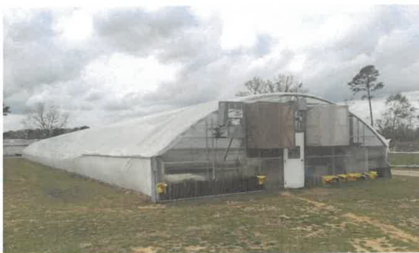
Figure 13: Greenhouse with Flexible Sides and Removable “Roof”
