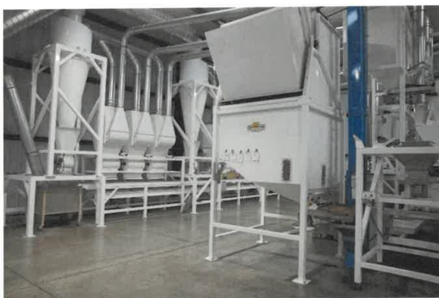
Figure 10: Structure Used for Processing Nuts
