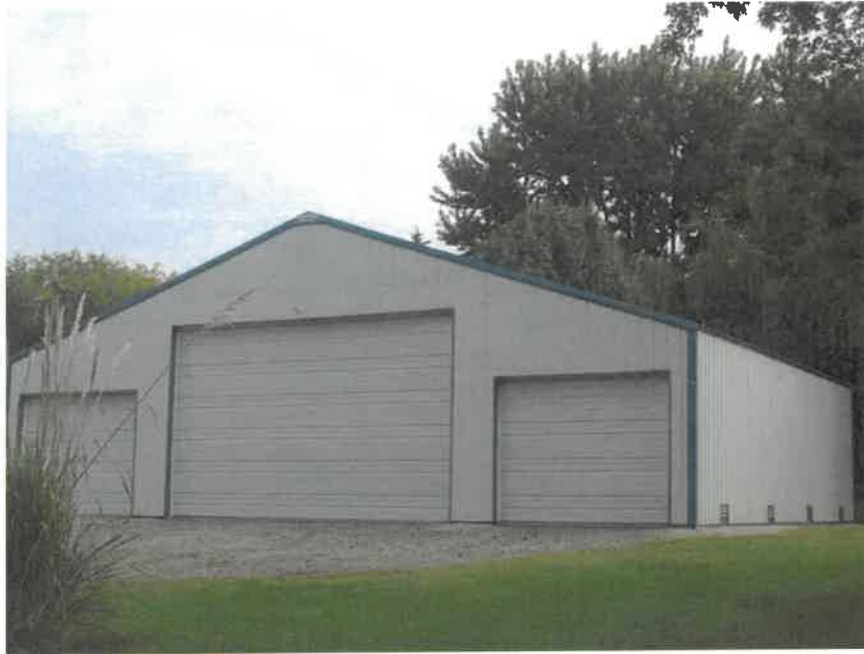
Figure 2: Agricultural Structure for Equipment and Storage, with Flood Openings (Source: Steve Samuelson, Kansas NFIP Coordinator)
