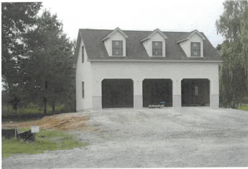
Figure 21: Three-Car Garage Elevated on Fill
