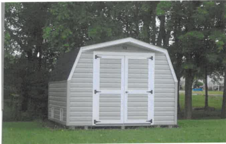
Figure 15: Storage Shed, with Flood Openings (Source: Kevin Wagner, Maryland Department of the Environment)
