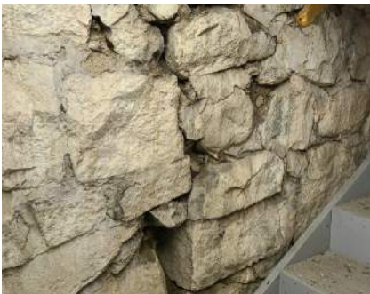
Foundation wall-basement entrance
