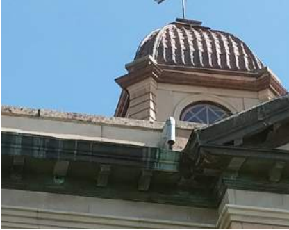
Dome and high roof gutter downspout
