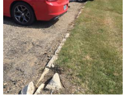
Damaged curb
