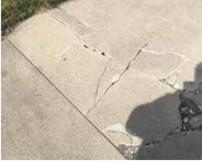
Cracked concrete panels
