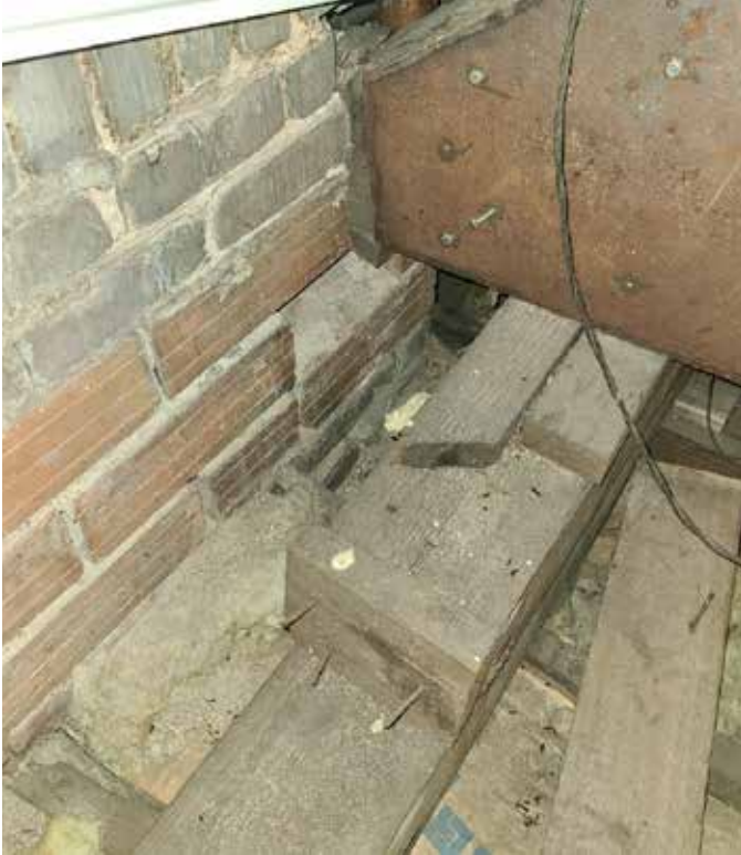
Northeast roof truss bearing—attic
