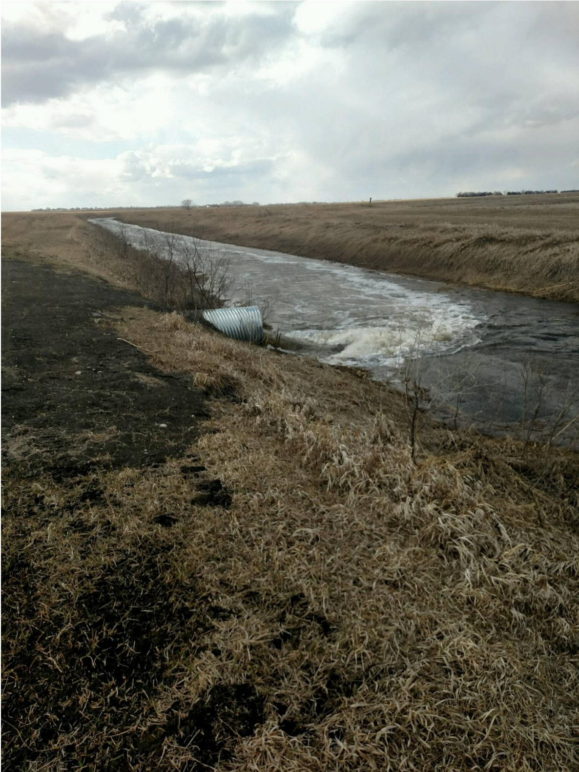
This picture is of the culvert which enters into the Wild Rice.
